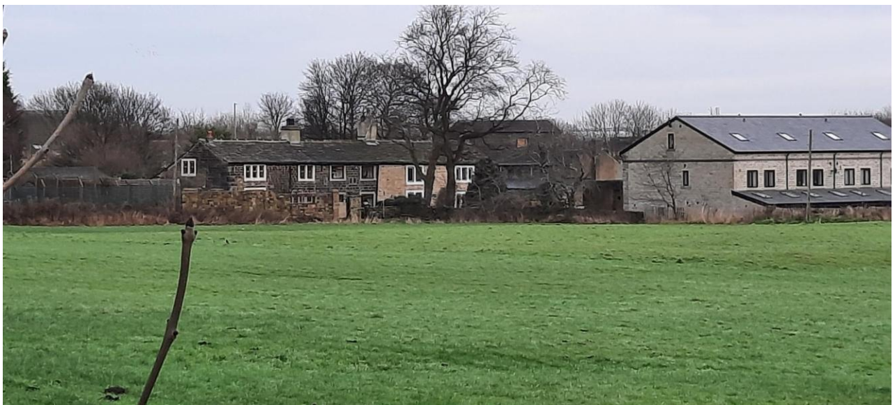
View of the south elevation of 1, 2 and 3 Abb Scott Lane from within the site
