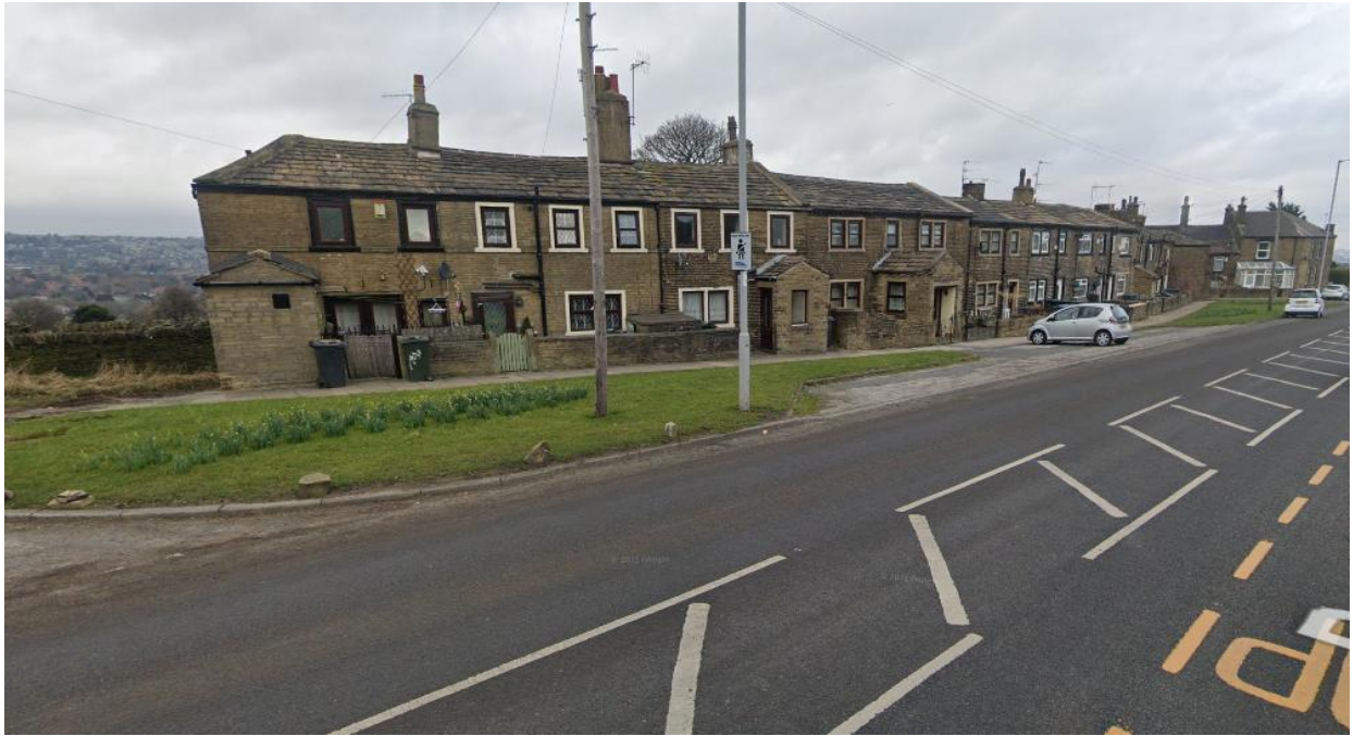
Photo 3: Nos. 152-164 Bradford Road (Grade II) (Image from Google Streetview)
